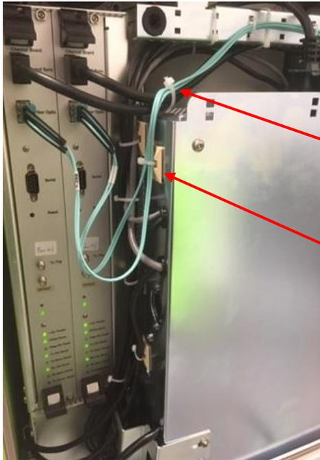
Figure 100: Sample Use of Cable Ties
